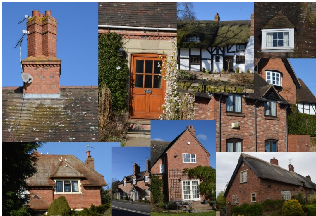
Figure 3 – 2 to 2.5 storey elevations of traditional red brick and timber frames, steep pitched roofs of red / brown tiles and thatch, and wooden door and window frames characterise residential development in Leek Wootton
