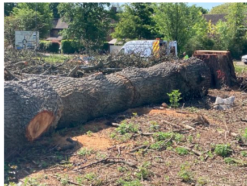
Photo above Leamington Road, Kenilworth to make way for 550 homes - 16 May 2022
